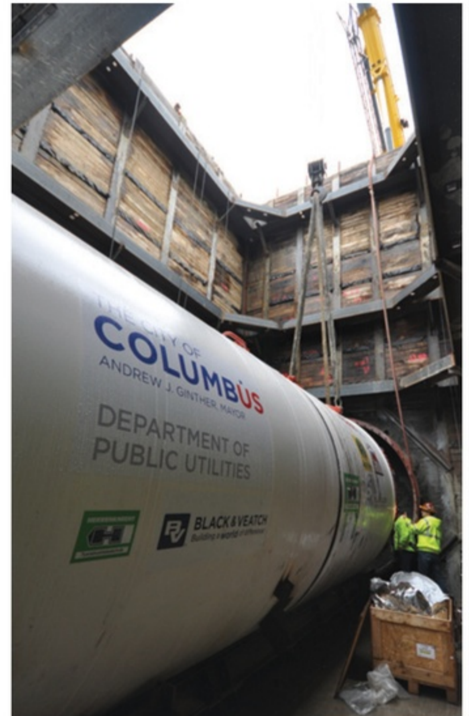
The TBM being lowered and readied for launch in the starter shaft
