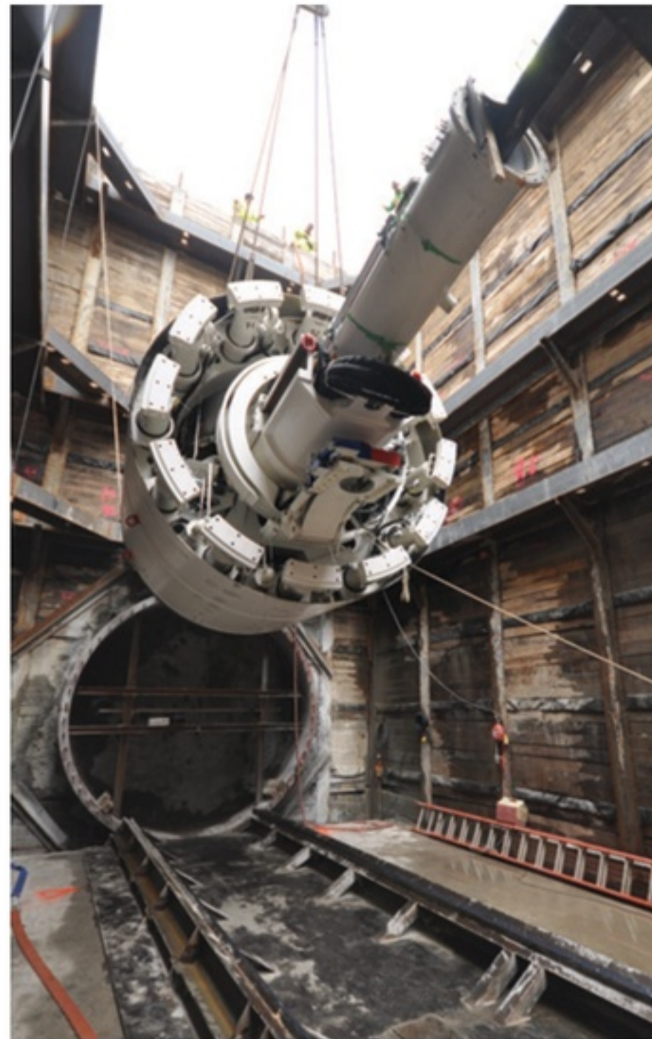
The TBM being lowered and readied for launch in the starter shaft
